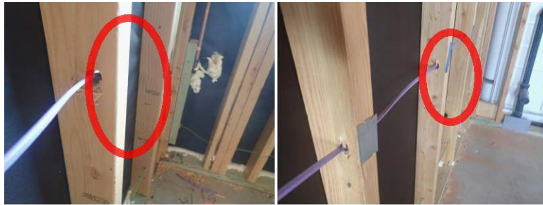
Missing nail plates
