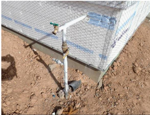
Main water line & valve
